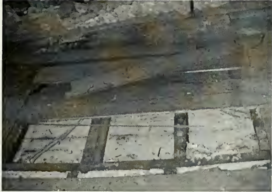
Figure 10 Opening for original Winder Stair, 2002
